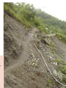
Landslide in Cascade Jamaica. Photo: Jamaica Conservation and Development Trust.
